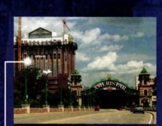
Ameristar Casino in St. Charles , a 26 story high rise with a large footprint, almost 300 by 100 feet, utilizing approximately 600,000 utility size bricks and approximately 75,000 square feet of glass fiber reinforced concrete, used Hohmann & Barnard's Flex Flash, a 40 mil self-adhering membrane.
