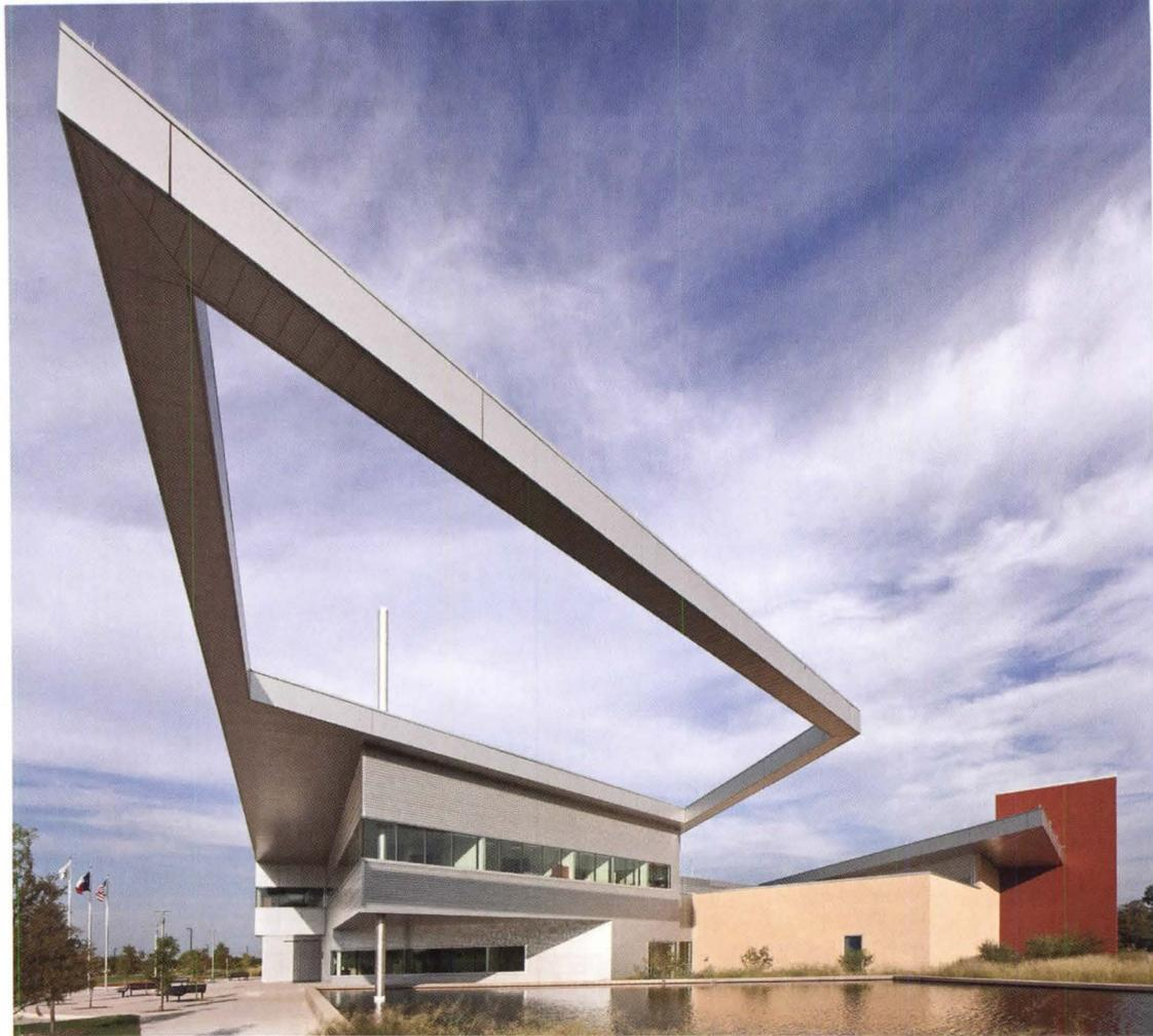
The construction of the 50-foot-long projecting roof on the new Perkins+Will-designed Public Safety Building in Lancaster, Texas, was not without its nail-biting moments. The entire steel assembly for the double cantilever was manufactured off-site and installed using supports. Once the welds were complete and the post-tension cables secured, the supports were removed and the cantilever was allowed to settle into place.
