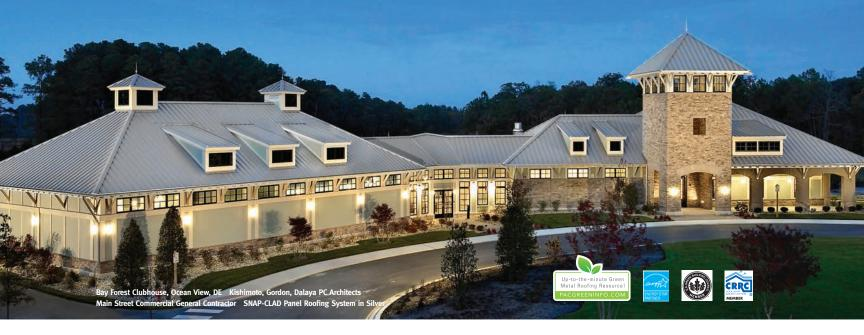
SNAP-CLAD<sup>™</sup> is available in 37 colors on aluminum and steel. Most colors meet LEED<sup>®</sup>, ENERGY STAR<sup>®</sup>, and cool roof certification. Also available with eave notching, for a properly trimmed eave detail and labor savings.
