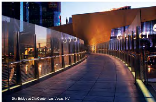
Sky Bridge at CityCenter, Las Vegas, NV
