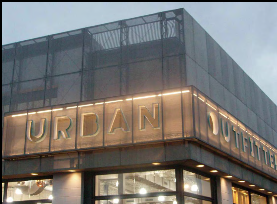
The trendy signage for the Atlanta Urban Outfitters store in Atlanta, GA, is made with McNichols® Designer Wire Mesh.
