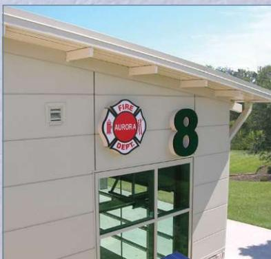
**Metl-Span ThermalSafe® panels combine maximum fire resistance with efficient, single-step installation.**
