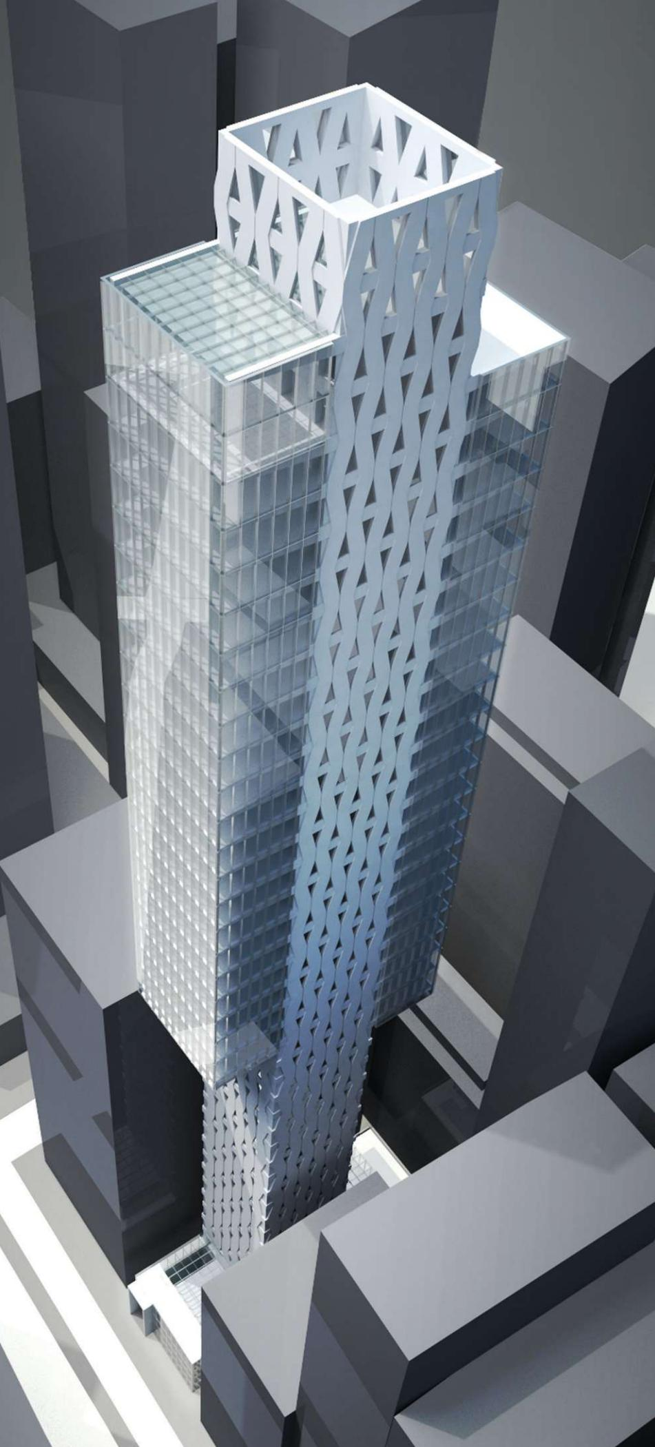
The concept of a structural core with cantilevered floor plates is by no means new, but extrapolating that technology to create high-rise towers, ranging from the 25-story tall Takshing House Redevelopment in Hong Kong (left) to the 110-story Fluidic Tower in Seoul, South Korea (this image), to the 3,281-foot-tall a(Spire) Tower (far left) is the focus of SOM's research.
