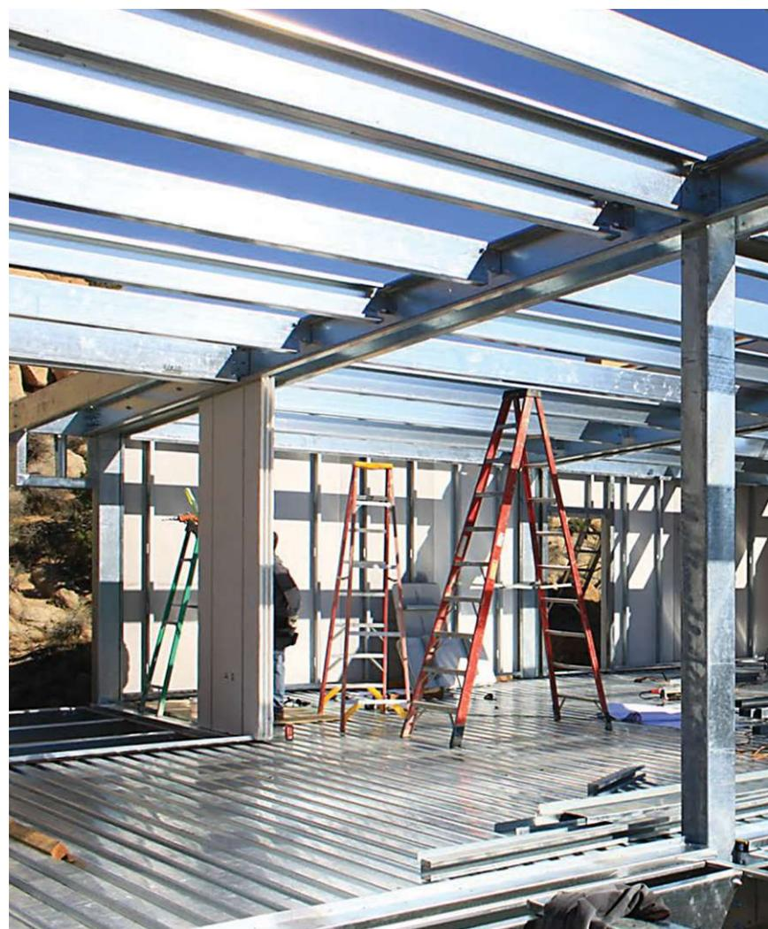
The Blue Sky Frame is lightweight enough to be assembled with minimal machinery and a small construction crew, and because it connects to structural concrete footings, it is minimally invasive to the landscape. The pregalvanized components are delivered and assembled without special equipment or tools, and a 1,000-square-foot house can go from bare site (top left) to nearly completed enclosure (bottom right) in as few as three days.
