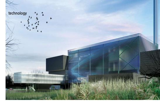
For the Sita UK waste-to-energy plant near Ipswich in Suffolk County, England, architecture firm Grimshaw was able to organize the various technical components and systems to create a more aesthetically pleasing massing than most WTE plants. Torqued louvers reflect natural light, and a transparent skin allows visitors to peek inside to catch a glimpse of the workings of the energy-production process.
