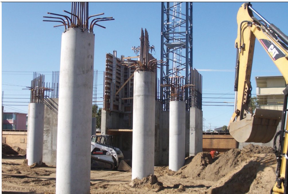
Column forms are often placed around reinforcing steel before concrete is pumped into the forms. After the concrete has set, the form is removed.
