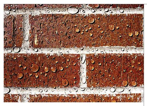
Rainwater penetration is caused by the presence of water on the substrate, openings in the substrate that allow water penetration and/ or pressure differences that drive water through the structural backup.
