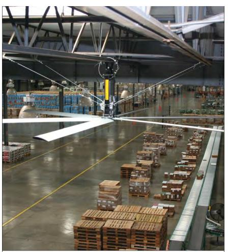
HVLS fans can range from 8 feet in diameter to 24 feet in diameter and can circulate more than 500 cubic feet of air per minute. (photo courtesy of MacroAir Technologies)
