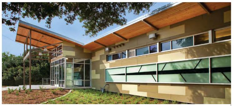
Common rainscreen claddings include: brick veneers, stud back-up, stucco, clapboard, panelized wall systems such as metal, alpolic, and fiber cement.
