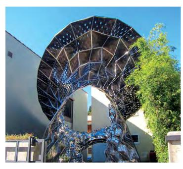
The Bloom pavilion, designed by Doris Kim Sung, is composed of panels made of two different types of metal that curl at different temperatures.
