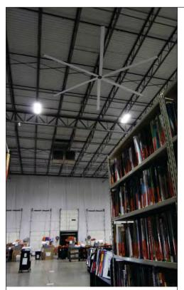
Obstructions, like the shelving pictured here, can greatly reduce the effectiveness of air movement generated by fans. However, larger downward air columns and deeper horizontal floor jets can overcome obstructions at floor level.
