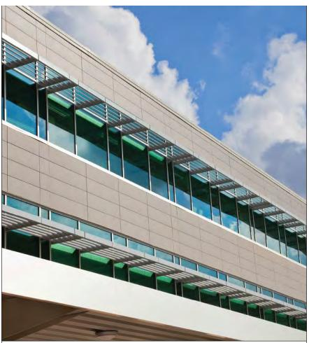
Moisture intrusion in a wall system can be the cause of building defects, as well as health ailments for the building's occupants, making rainscreens a very important tool in water mitigation.
