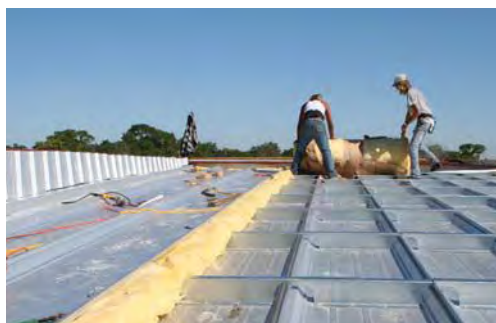
The cavity between the old and new roofs can be used to add insulation. Photo Credit: Roof Hugger
