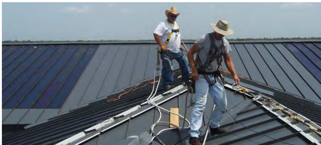
The decades-long service life of standing seam metal roofs makes them ideal for rooftop solar installations. Whether with crystalline photovoltaic arrays or thin film laminates (as pictured here), metal allows PV systems to be installed without creating roof penetrations. Photo Credit: Drexel Metals
