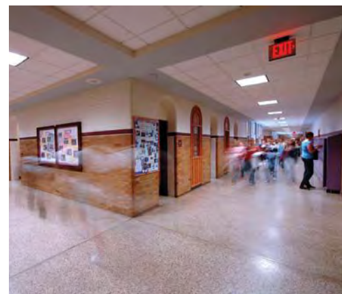
The tough, flexible finish of high performance acrylics makes them a good choice for high-traffic areas like school hallways and stairwells, where they can withstand abrasion while maintaining an attractive finish. Photo Courtesy of Sherwin-Williams
