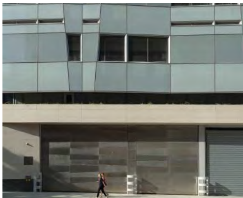
The Belfer Building's undulating south facade controls solar thermal gain passively with a double curtain wall whose perforations let warm convection currents escape the cavity between its inner and outer surfaces. © Tex Jernigan
