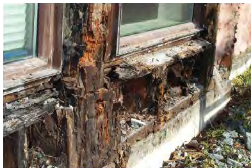
Internal moisture degradation is a leading cause of premature failure of building envelopes. Photo courtesy of Cosella-Dorken
