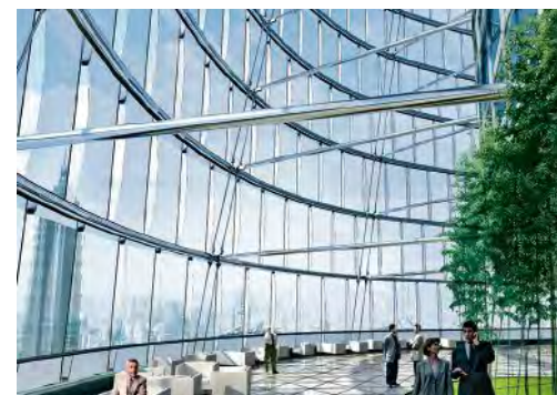
The building skin is suspended from above on huge cantilevered trusses that are stabilized by hoop rings and struts. © Gensler
