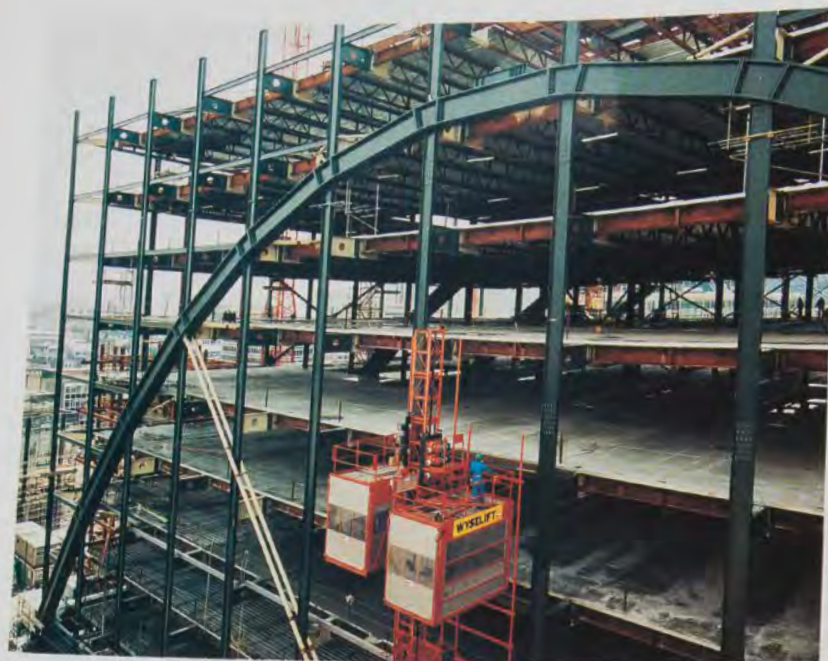
Floor trusses span the bays within the building and connect either to girders or directly to the exterior columns. The arches are constructed of parallel steel channels (above) with an intermediate space to allow the columns to pass through the arch (facing page, top left).
