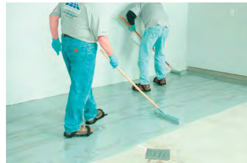
Polyaspartic coatings are typically used where there is fast return to service time desired, as they cure very quickly. Photo Courtesy of Bayer MaterialScience
