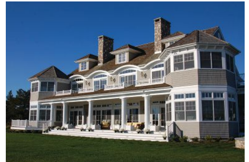
Some advantages of cellular PVC materials over wood trim are that it won't rot, it resists insect infestation, and it can be placed in direct contact with the ground, masonry or even direct moisture. Photo courtesy of VERSATEX Trimboard
