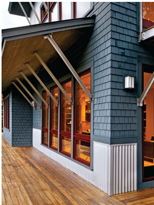
Not all paints require a primer coat or clear coat, but bright colors such as red often require a top coat.
