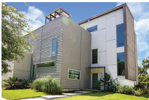
Extruded aluminum adds durability and longevity to construction that other trim materials such as galvanized steel and polyvinyl chloride (PVC) lack.
