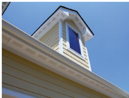
Cellular PVC does not require painting for protection, but can be painted to achieve a custom appearance. Photo courtesy of VERSATEX Trimboard
