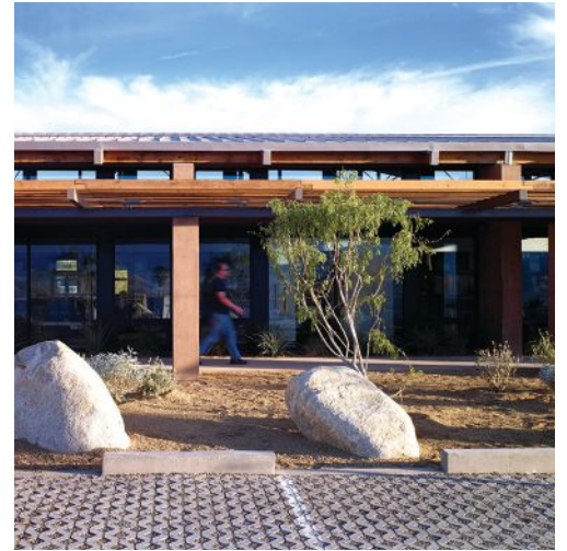
Extended wooden trellises form a shaded outside perimeter, helping manage solar gain and limiting interior cooling and lighting expenses.
