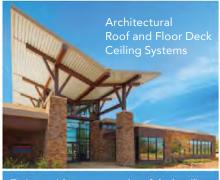
Toris provides a structural roof deck ceiling or soffit that clear spans up to 30 feet with options that can include superior acoustics, hanging features, and access panels.
