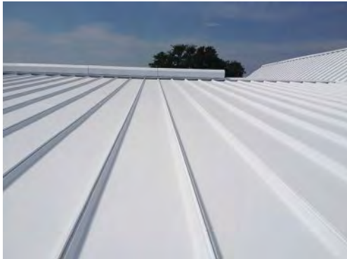
Reflective coatings are often applied over darker colored or aged reflective existing roofs to help reduce energy costs.
