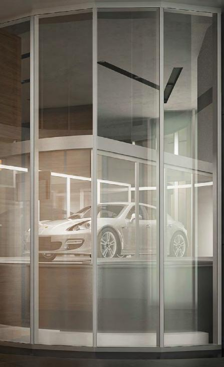
2 HOUR FIRE RESISTIVE GLASS INTERIOR/ELEVATOR ENCLOSURE WITH SUPERLITE II-XL 120 IN GPX CURTAIN WALL FRAMING
