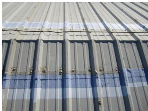
The surface must be exceedingly clean, and seams and penetrations must be properly prepared. Photo courtesy of Neogard, a part of the Hempel group
