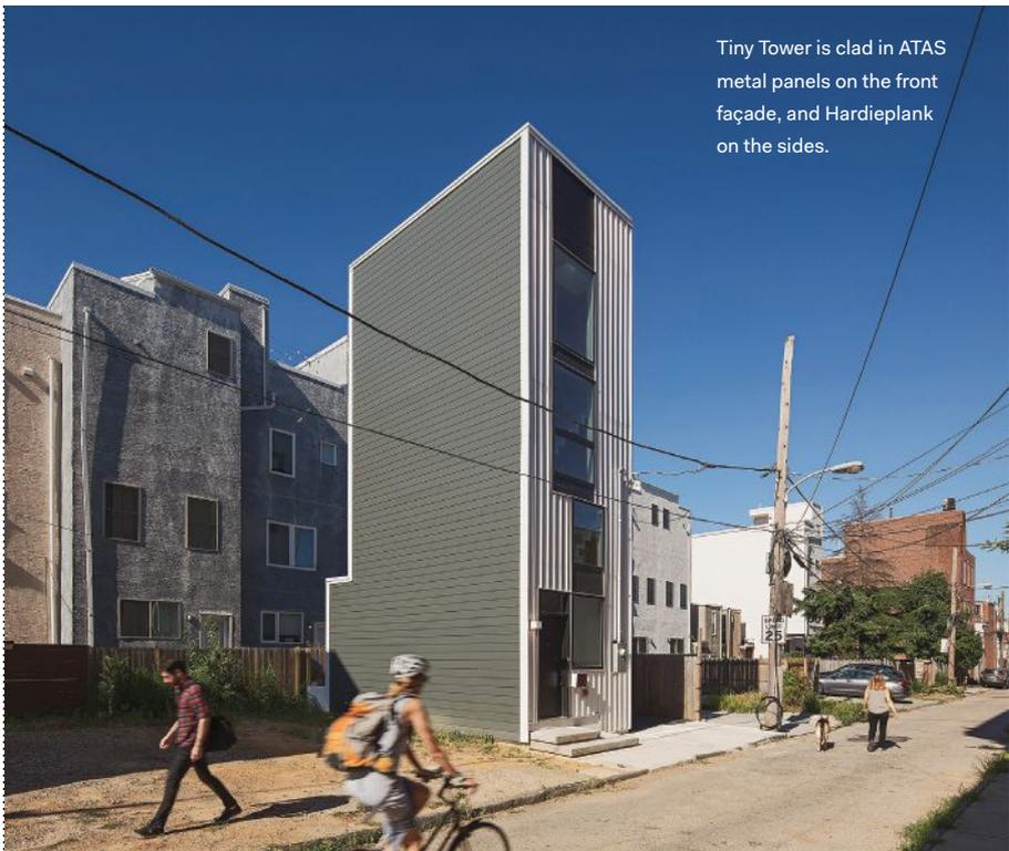
Tiny Tower is clad in ATAS metal panels on the front façade, and Hardieplank on the sides.
