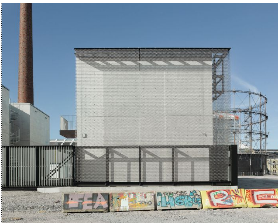
The new substation has site-poured concrete walls with a Codina Architectural stainless steel mesh overlay.
