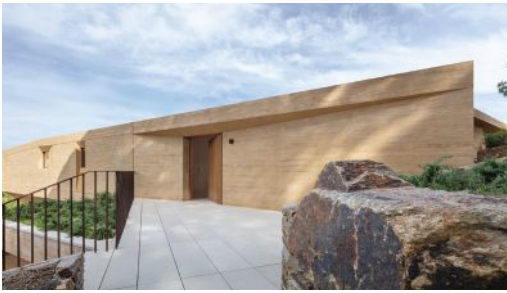
The main entrance sits at the west corner of the house.
