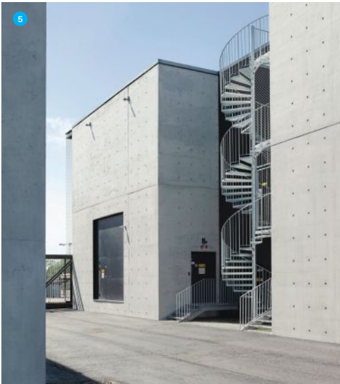
1. The concrete, from Rudus Oy, has titanium oxide in the mix to give it a whiter tone. 2. A nearly 10-foot-high blank aluminum fence surrounds the substation on three sides, purposefully providing a canvas for local artists. 3. The building interiors, which are kept largely confidential for security purposes, contain equipment that is part of a new, district-wide smart grid. 4. The substation sits directly next to the decommissioned 1909 Suvilahti power plant, which has since been turned into a cultural center. 5. A central court between the structures, and behind the fence, allows for secure vehicle access for service.
