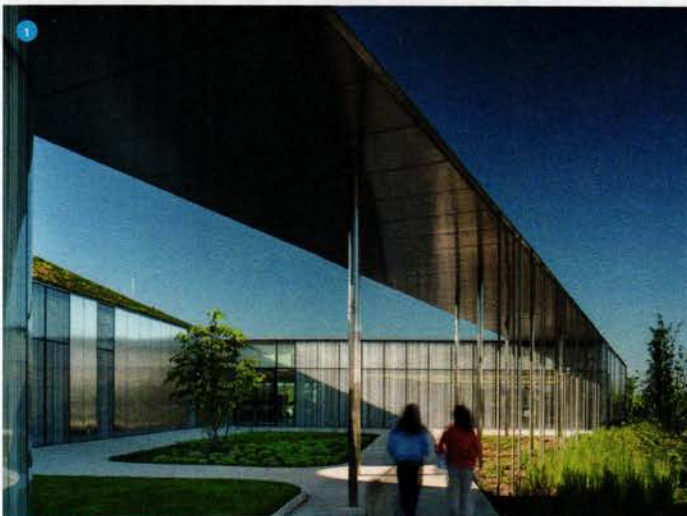
1. Super-thin steel columns help support a stainless steel canopy at the eastern edge of the building; a courtyard provides green space in front of the main entry (at center). 2. At the western edge of the site, terraced concrete walkways and benches with a series of pools create a buffer between the library and the street.
