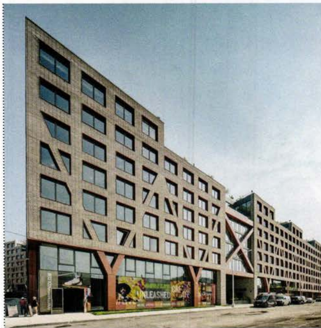
The north façade has retail at the base.
