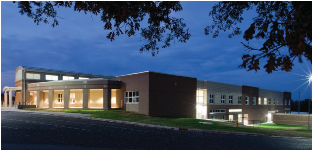
Richardsville Elementary School is the nation's first zero energy school. Photo courtesy of Sherman Carter Barnhart Architects.
