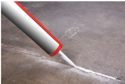
Since the main objective of a sealant is to seal assemblies and joints, sealants need to have sufficient adhesion to the substrates and resistance to environmental conditions to remain bonded over the required life of the assembly.
