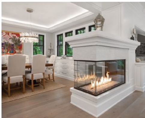
Power venting allows direct-vent fireplaces to be installed anywhere in the building, including interior walls and other central spaces.
