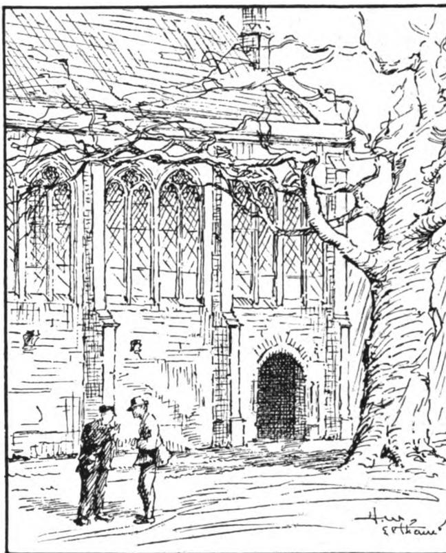
because it was useful as a barn, owing to its size, but the glass perished and the windows were bricked up. A century ago the roof-covering disappeared, and the rain had free access. The walls were never strong enough to hold the roof from spreading, and as this happened the windows were forced out of position. In this state the government took a hand, and, classing the hall as a national monument,
