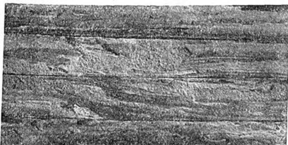
Damage to pine timber in building by the old house borer hylotrupes cajulus , a powder-post beetle which lays eggs under edgings of bark
