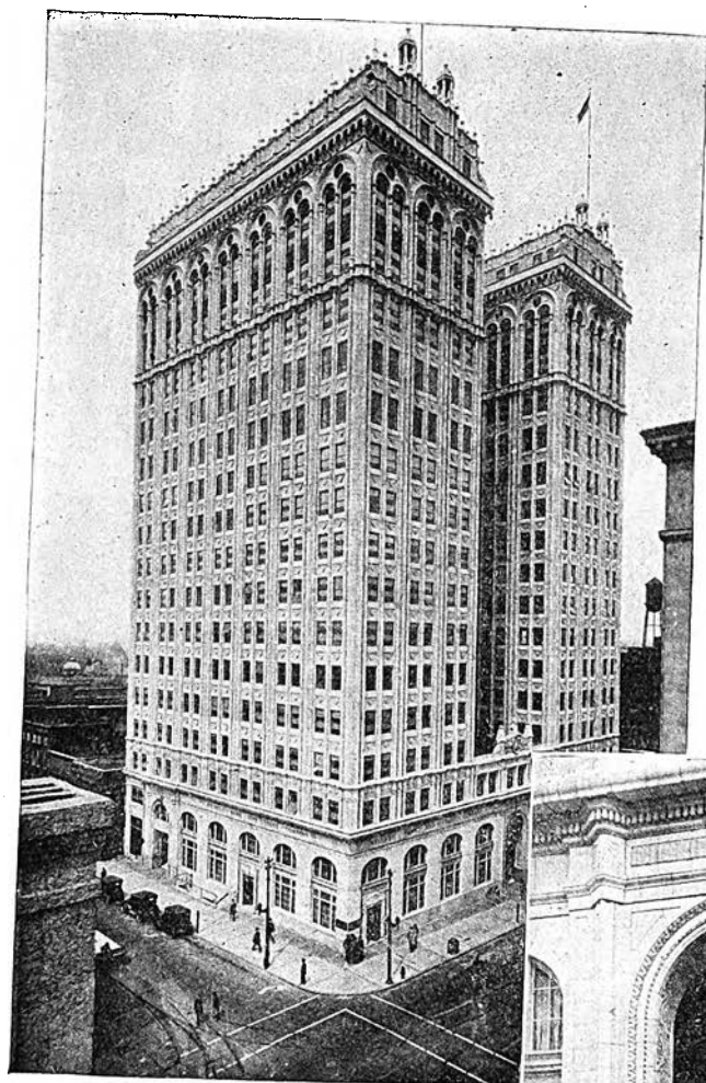
Jefferson Standard Life Insurance Company Building, Greensboro, N. C. Charles G. Hartman, Architect. Excepting base course and plain granite ashlar surrounding arched windows of lower story all exterior masonry material is unglazed granite colored Terra Cotta, including the arched entrances with their elaborate ornamental detail.
