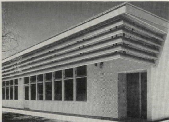
KAWNEER K-LOUVER —Rowland Union School, Puente, California. Lee B. Kline, A.I.A., Foster Simpson, Illuminating Engineer.
