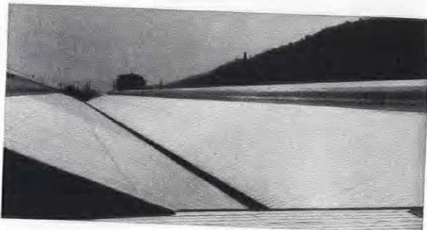
Roofing and Roof Decking
