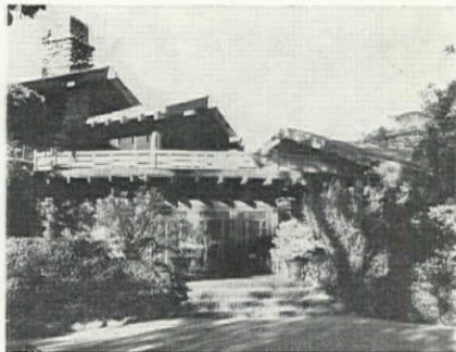
13 Charles Pratt House, Ojai, California. Entrance detail
