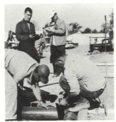
Placing of floor heating ducts
