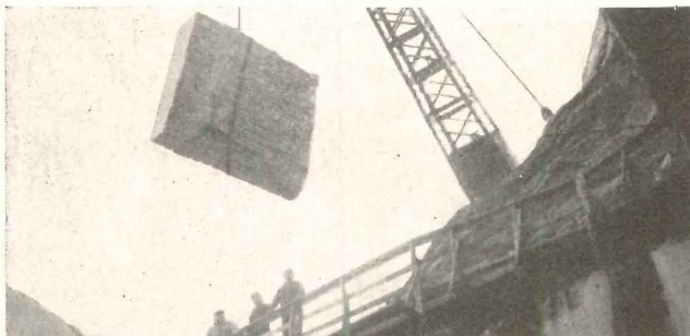
Outsize blocks of marble were taken from our Danby quarry for this installation. 250 slabs with random, non-matched veining were specified by architects Skidmore, Owings & Merrill.
