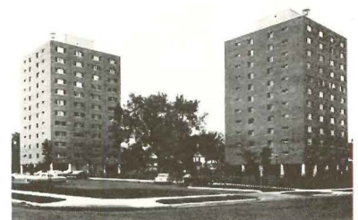
Elliot Twin Apartments, Minneapolis. Architects: Thorsen & Thorshov, Inc.
