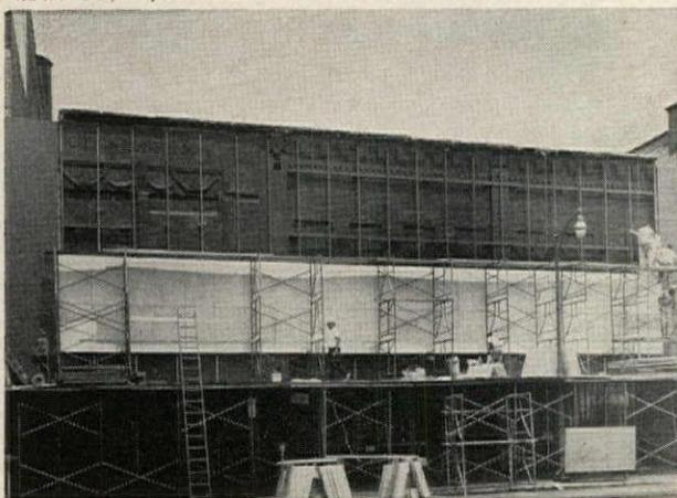
In remodeling work, the Zibell struts simply bridge over the projections and recesses in the old wall, obviating much costly remedial work. A Zibell installation is comparatively
