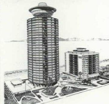
**Tower Apartments, Long Beach, California:** Carl B. Troedsson, architect; T. Y. Lin & Associates, structural engineers. Central core enclosing elevators (visible at top of construction photo) was slip-formed first, then surrounded by a circle of steel columns tied to the core by post-tensioned floor slabs. The 34-story tower, tallest prestressed concrete building to date, is designed for high earthquake resistance.
