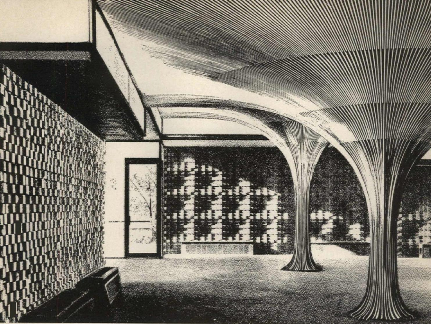
Plastic forms were used for precision casting of these columns. The high-early-strength concrete, made with Lone Star's INCOR® 24-hour portland cement, permitted forms to be stripped the following day. Maximum aggregate size was 3/4".
