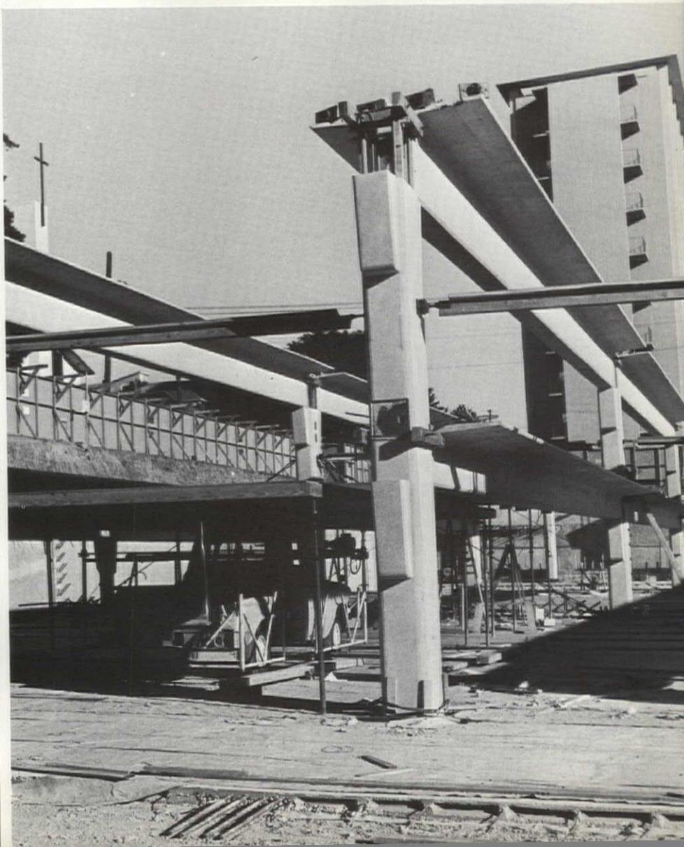
**University of California Office Building, Davis:** Gardner A. Dailey FAIA, architect; T. Y. Lin, Kulka, Yang & Associates, structural engineers. Entire building used essentially three types of precast components — nine-story columns (each cast in one piece), two-story wall panels and channel-shaped floor sections. Grooves in wall-panel sections were used for visual interest. Building, 36x127 feet, contains no beams, girders.
