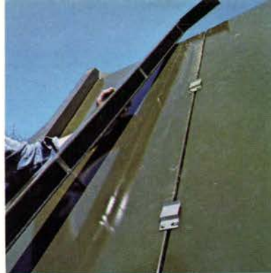
Raised channels simply slip into brackets to cover joints.
