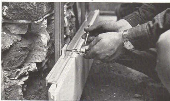
Horizontal members fastened by special clamps.
