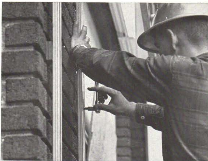
Vertical struts are anchored to existing facade.
