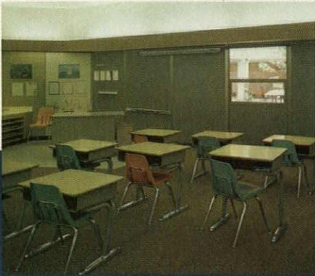
Versatile Mirawal insulated panels are ideal for modern school use—one panel can serve as the complete wall with porcelain enamel on both the outside surface and the floor-to-ceiling chalkboard inside.
