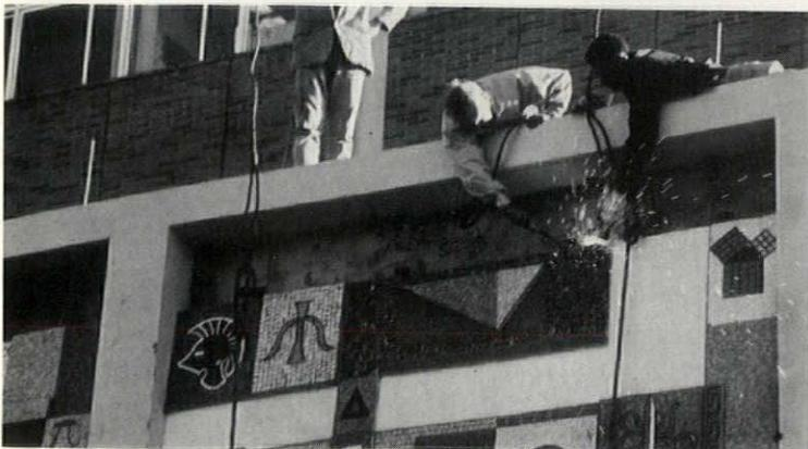
Installation team cuts supporting cables, then threads panel in position with lifting cables lined up with precast grouting holes on the roof. The mosaic pieces are in hundreds of colors.
