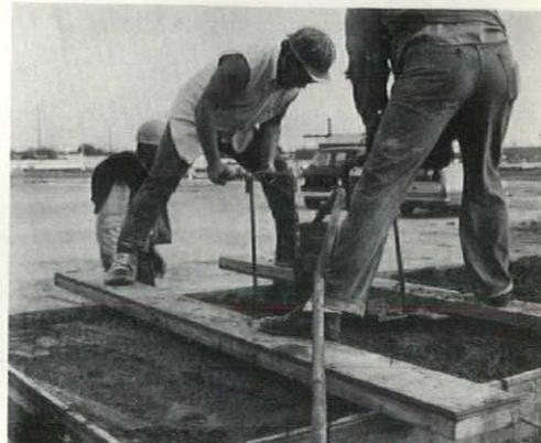
Third and final level of concrete is compacted. After overnight curing, panels are hoisted onto A-frames for cleaning and storage.
