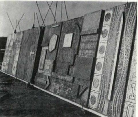
Panels, resting on A-frames, in various degrees of the cleaning process. Two sets of lifting cables were cast into each panel.
