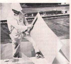
Pre-formed parts of Type 304, 26 gauge JaITEX stainless steel were delivered to the site by the mechanical contractor.
