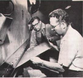
Pre-forming JalTEX stainless steel sheets at the Temp-Control Corp. plant. Edges for joining were crimped one-half inch for flat-seam joining.
