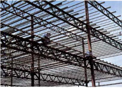
The simplicity and light weight of Vulcraft joists and joist girders make erection fast and easy.
