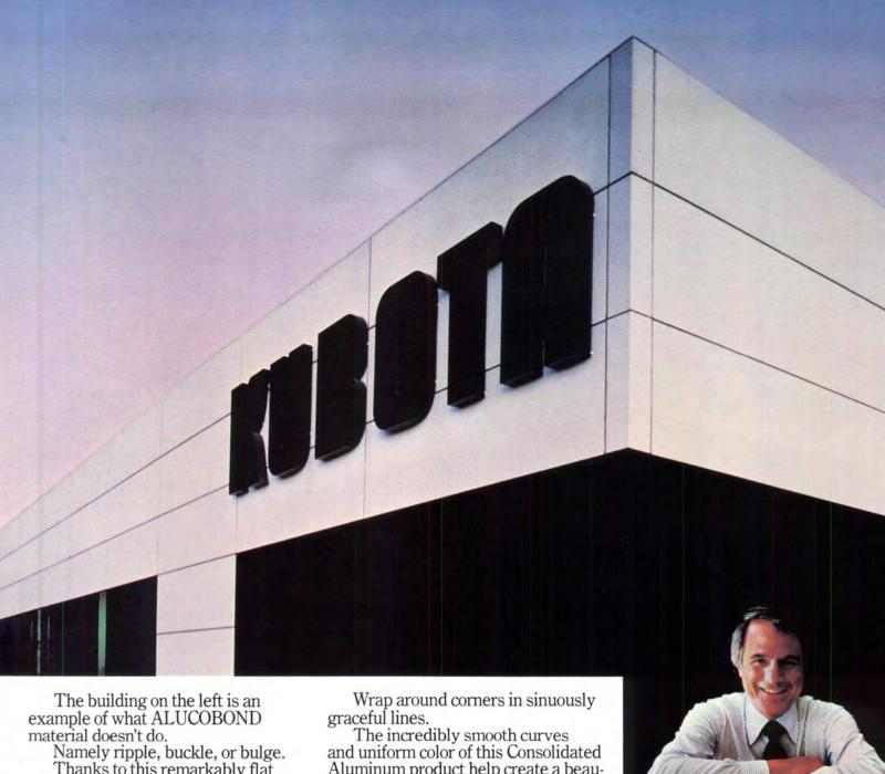
Namely ripple, buckle, or bulge. Thanks to this remarkably flat composite of two aluminum sheets and a thermoplastic core, oil-canning has been totally eliminated on Kubota Tractor's streamlined U.S. headquarters in Compton, California.
