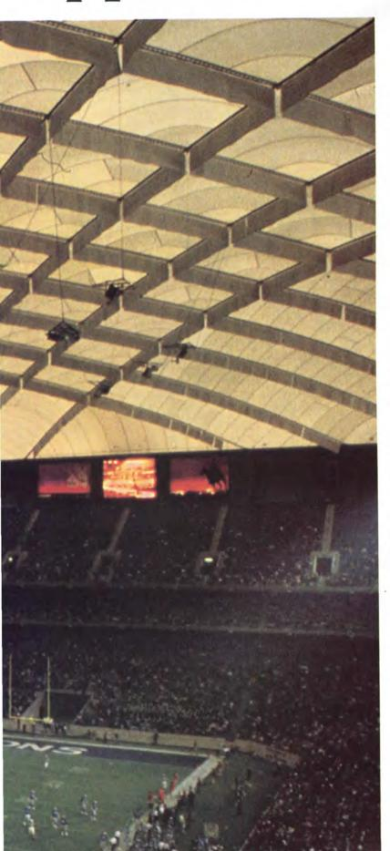
An air-supported dome of lightweight Fiberglas® coated with DuPont TEFLON® fluorocarbon resin completely roofs Pontiac Silverdome, home of the Detroit Lions, Detroit Pistons and Detroit Express. The 10-acre area is the largest permanent structure roofed with architectural fabric to date—and the stadium cost far less to build than comparable stadiums using other dome approaches.
