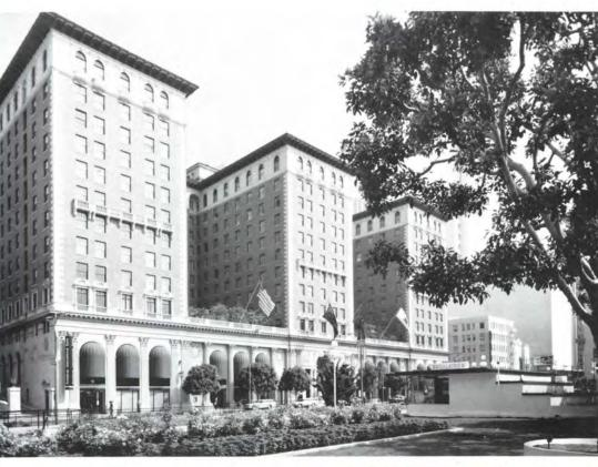
Restoration of the exterior (left) included tuck pointing, acid washing of masonry, epoxy injection on terra cotta and repair of wooden double-hung sash. On the interior (below) cast plaster was used for the repair of ornamentation.
