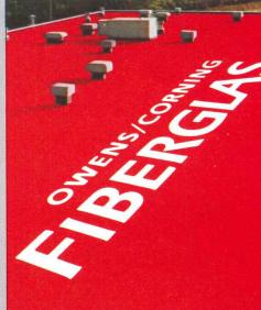
Perma Ply No. 28 base sheet. 2 plies Perma P No. 11. Perma Cap surface over wooden deck
