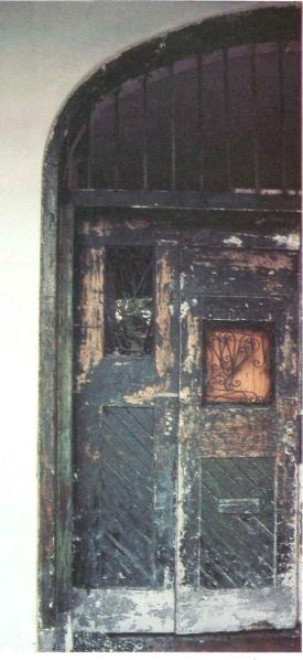
New Orleans is semitropocal, humid, frequently musty. Soil is the consistency of gumbo, and masonry walls draw its moisture. A lot of time is spent cleaning away mold and mildew. Paint jobs don't last very long, and things soon take on a patina, whether you want them to or not.
