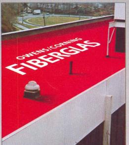
Double-layer Fiberglas insulation. 4 plies Perma Ply-R. Smooth surface.
