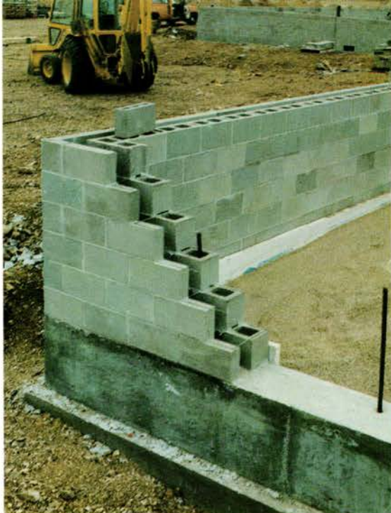
Cavity walls are of 8" concrete block with 4" block veneer. The cores were grouted. Cavities were filled with foamed-in-place insulation.
