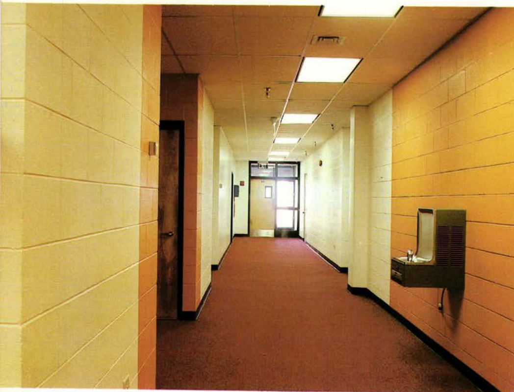
Interior walls of concrete masonry, used for thermal storage, are employed throughout the project.
