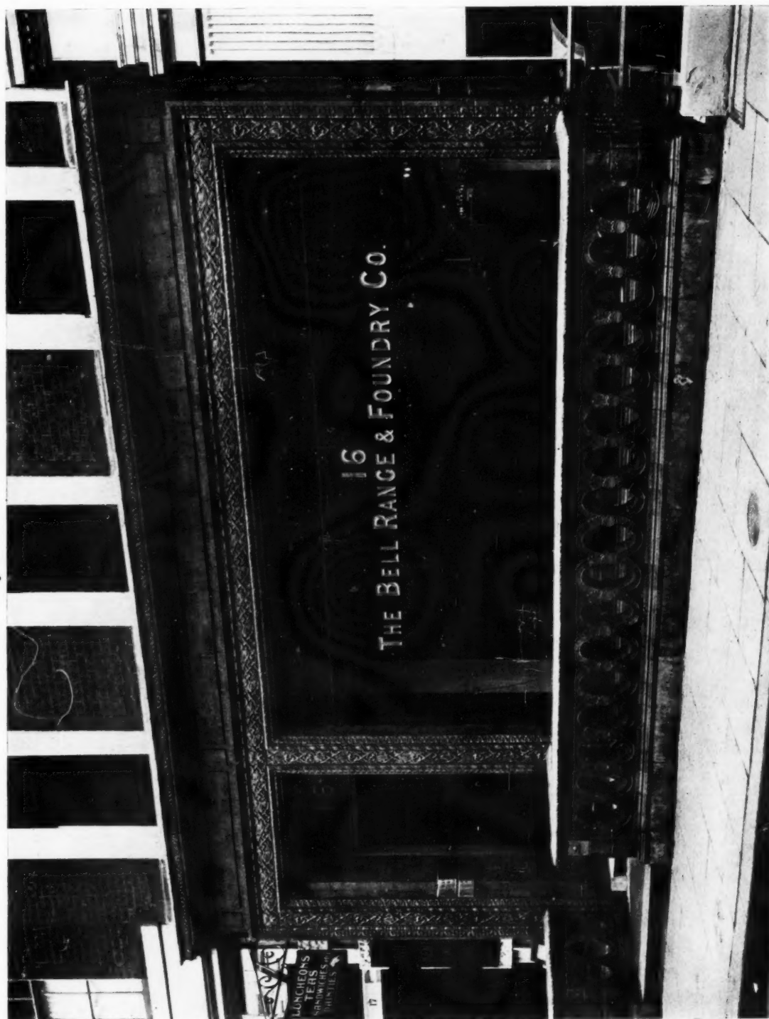
Faience is here effectively employed for the surround and balustrade of a shop front. The character of the detail is specially adapted to interpretation in that material. The colouring is indicated on the working drawing above.
