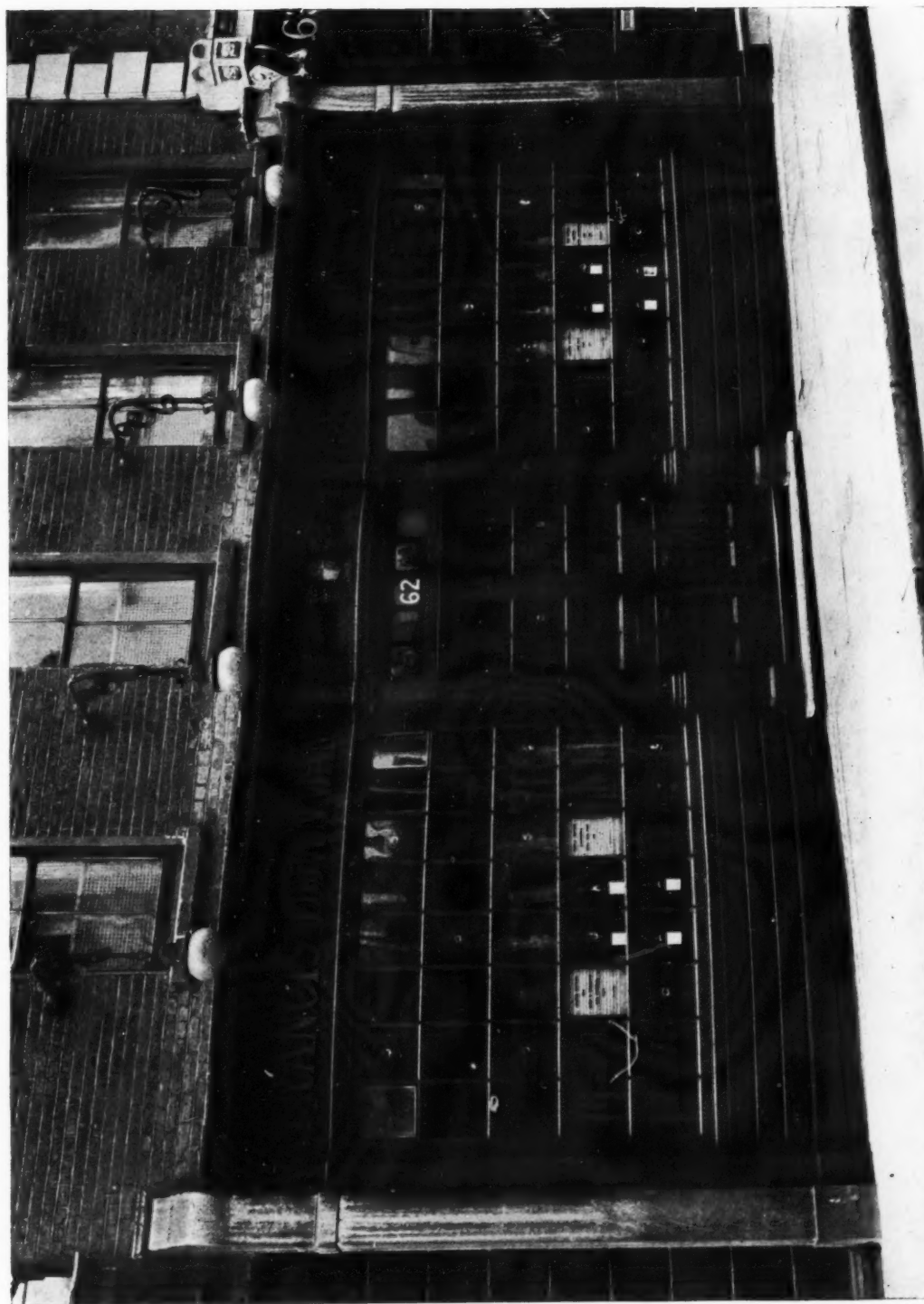
A successful attempt has here been made to fit an Early Georgian house with a shop front true to period. The front is of oak.
