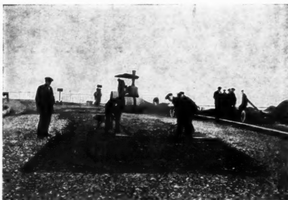
A REINFORCED TAR-MACADAM ROAD UNDER CONSTRUCTION AT REDCAR.
