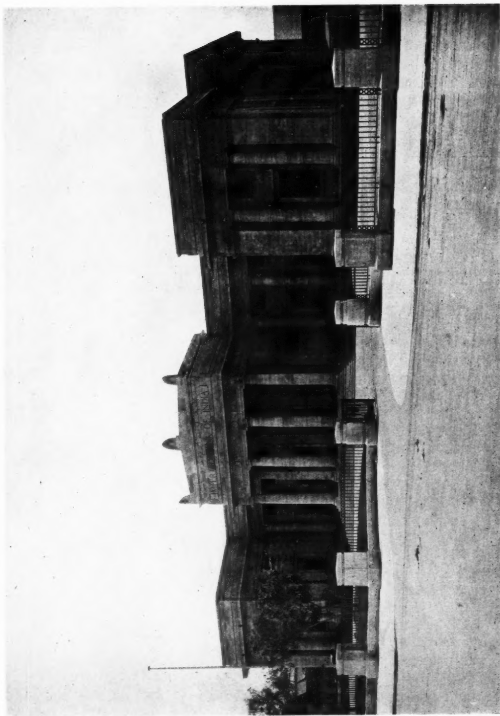
A recent example of Anglo-Indian architecture. Jodhpore pink sandstone is used for the exterior. The banking hall, which is entered through the portico and vestibule, runs the full length of the building, and measures 150 ft. by 50 ft. with a height from floor to ceiling of 28 ft.
