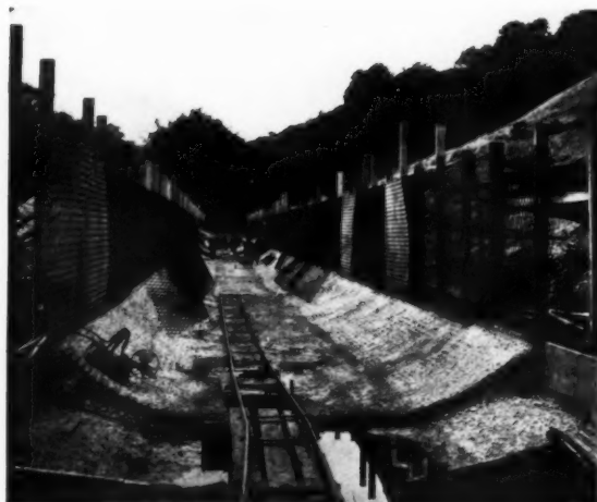
THE REINFORCED CONCRETE CULVERT UNDER THE NEW ROADWAY AT CASTLE EDEN, CO. DURHAM.
