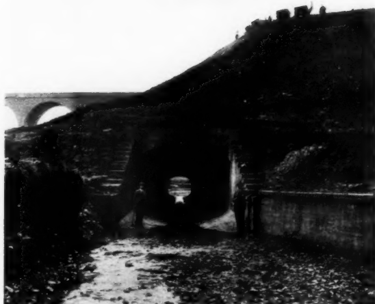
THE REINFORCED CONCRETE CULVERT UNDER THE NEW ROADWAY AT CASTLE EDEN, CO. DURHAM.
