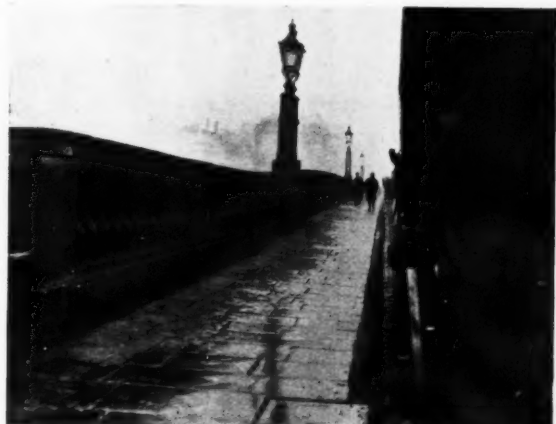
THE PARAPET, SHOWING FRACTURES AND SUBSIDENCE.
