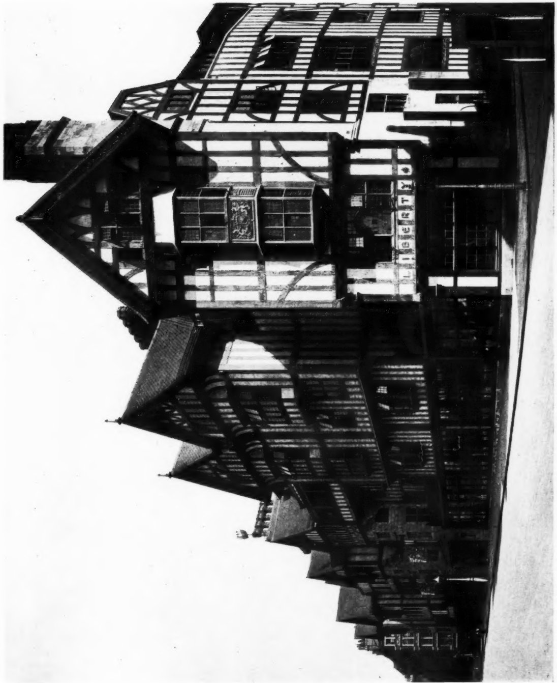
Messrs. Liberty's new building has been erected on a site on the east side of Regent Street, near Oxford Circus. The oak and teak used in the main structure came from H.M.S. "Hindustani," which was almost the same length as the main front.
