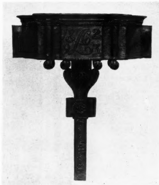
A CAST LEAD RAIN-WATER HEAD.
