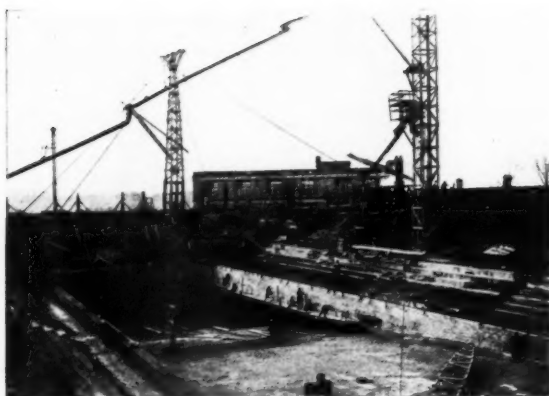
The "sheen" (left) joined to the high "sapine," used for the distribution of the concrete.
