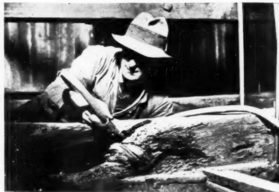
6. A large cross-beam eaten away by the death-watch beetle.
