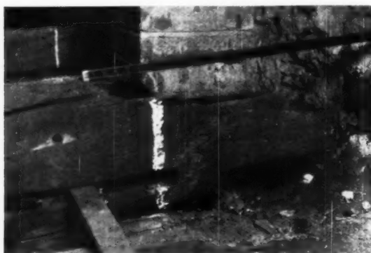
7. End of the main ceiling beam. White line shows bearing.
