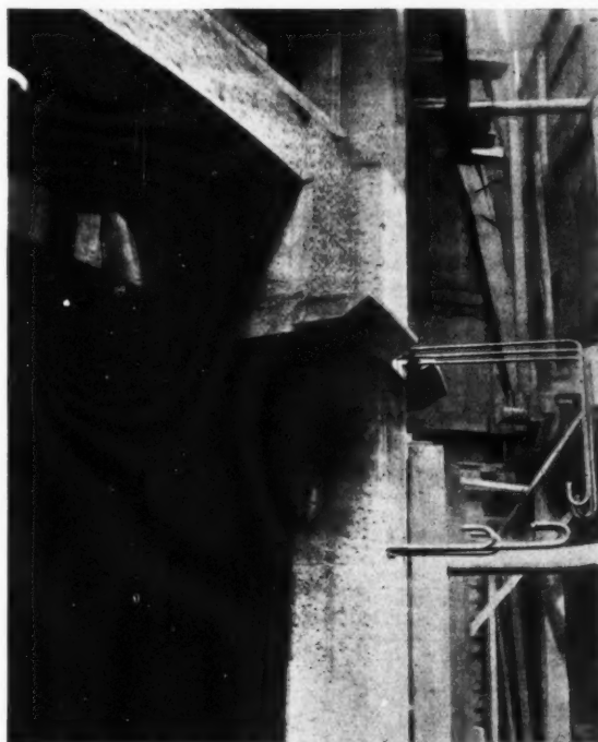
A detail of the reinforced concrete showing bracket to support ashlar facing.
