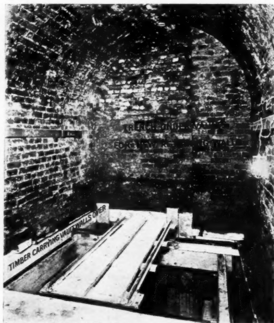
TRENCH UNDER VAULTS FOR NEW RETAINING WALLS.
