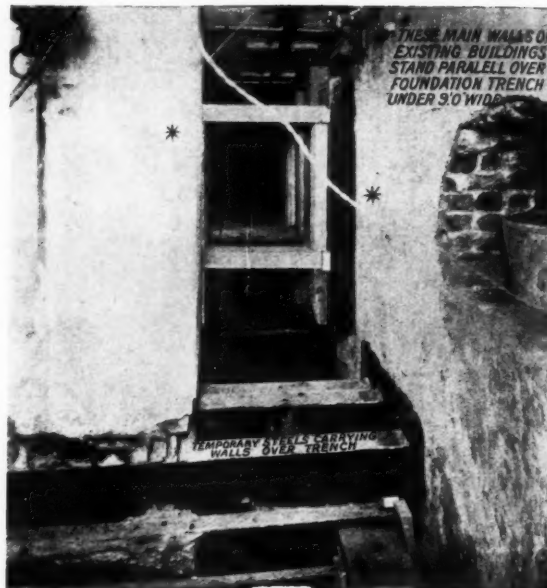
STEEL JOISTS AS TEMPORARY SUPPORTS FOR WALLS.
