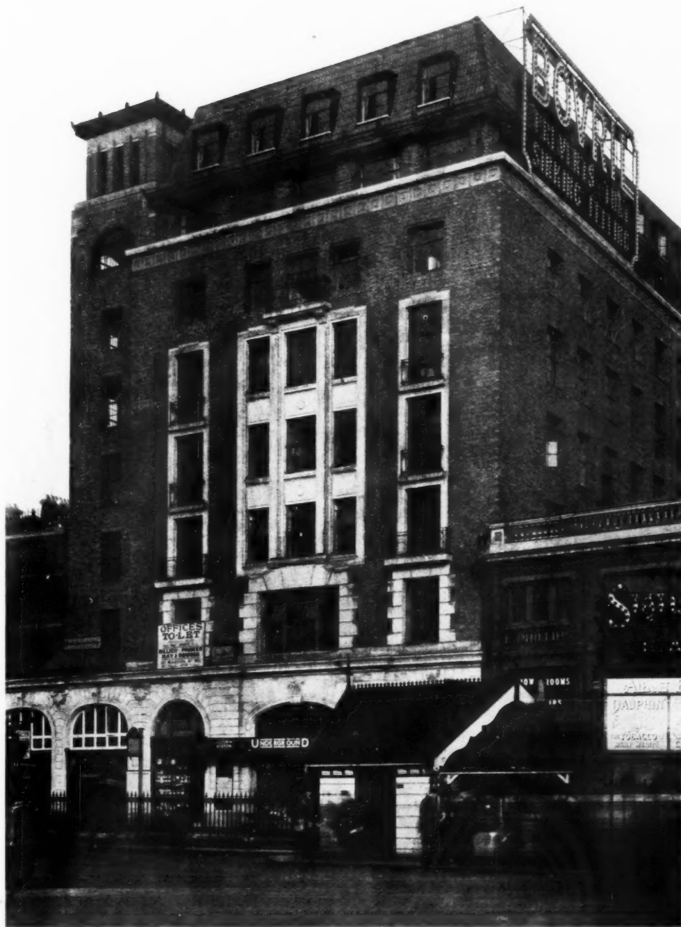
This façade faces the Victoria Southern Railway Station, just outside which the building is prominently situated. Multi-coloured bricks have been used for facing, and artificial stone for the parapet. The roof tiles are of Roman type.
