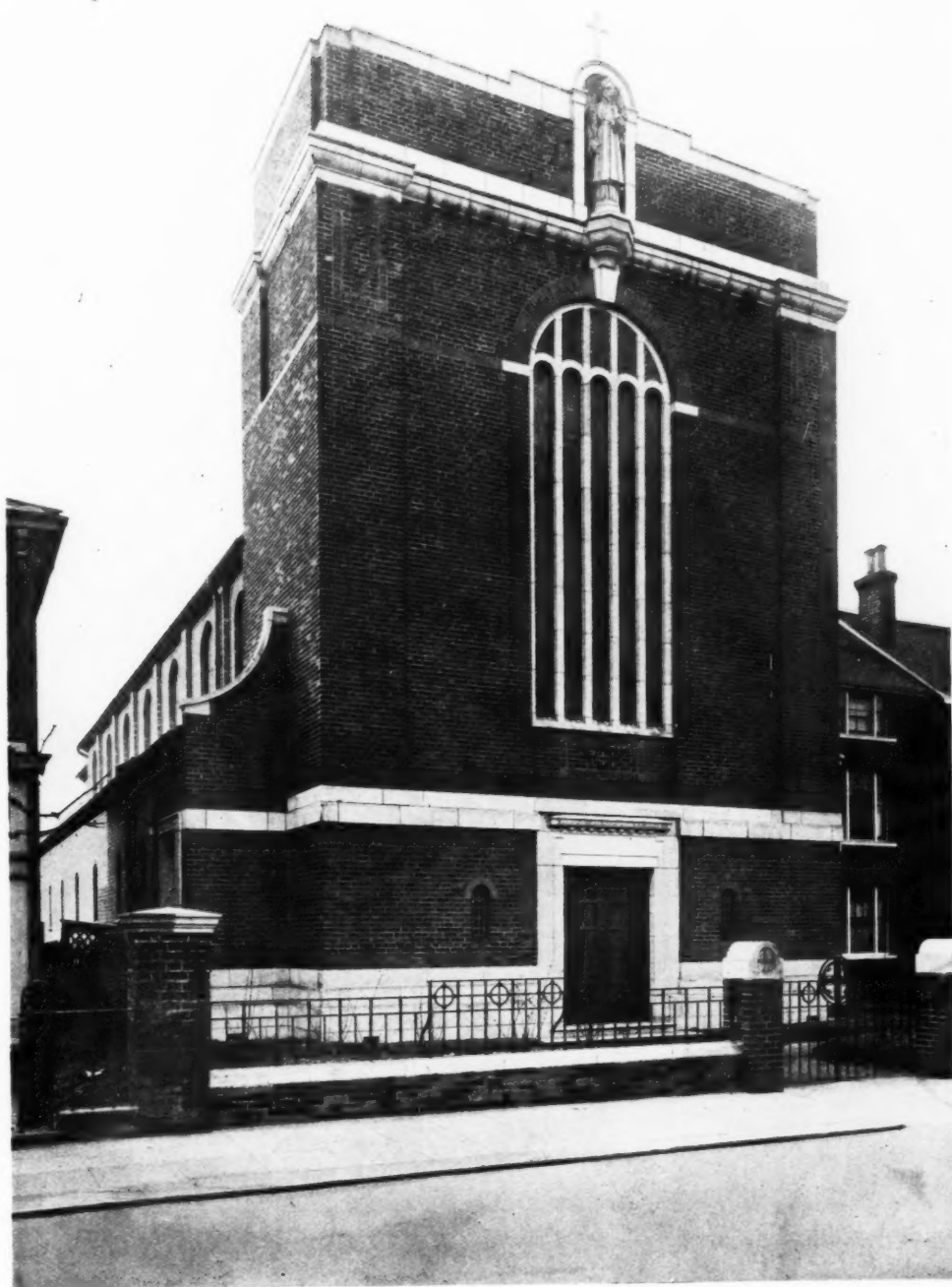
The whole of this church, except the brickwork of the tower and the side walls, is of steel-frame construction, with expanded metal reinforcement and plaster.
