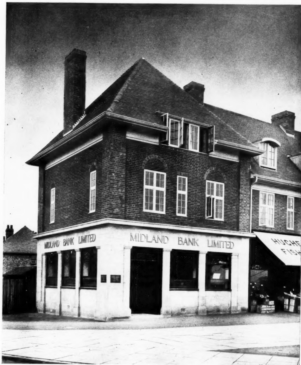
The elevations have been carried out with Titford and multi-coloured sand stock facings, and mottled Hollington stone and hand-made roofing tiles.
