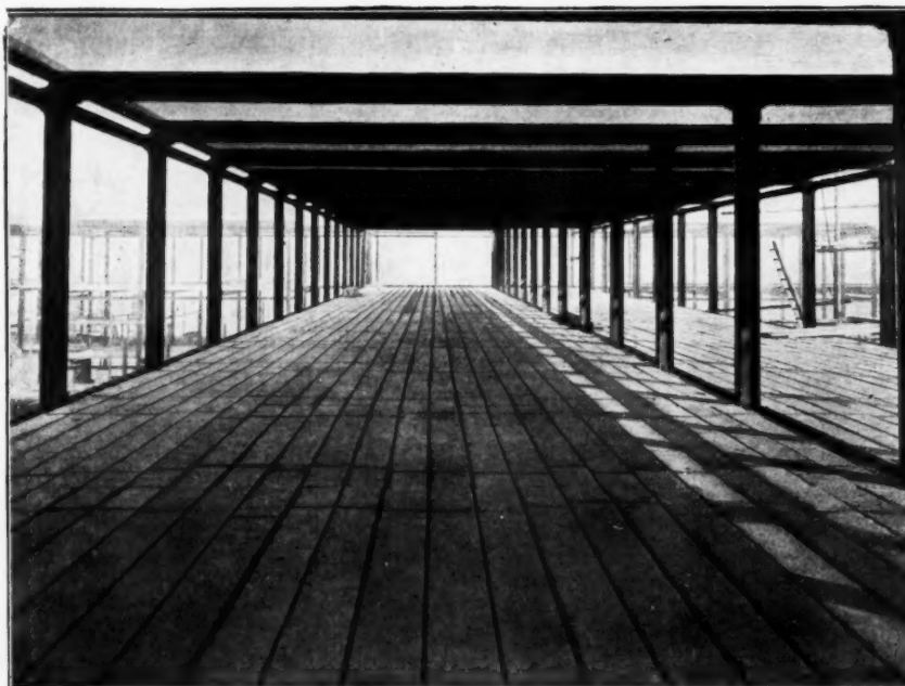
A CONCRETE FLOOR ERECTED ENTIRELY WITHOUT CENTERING
