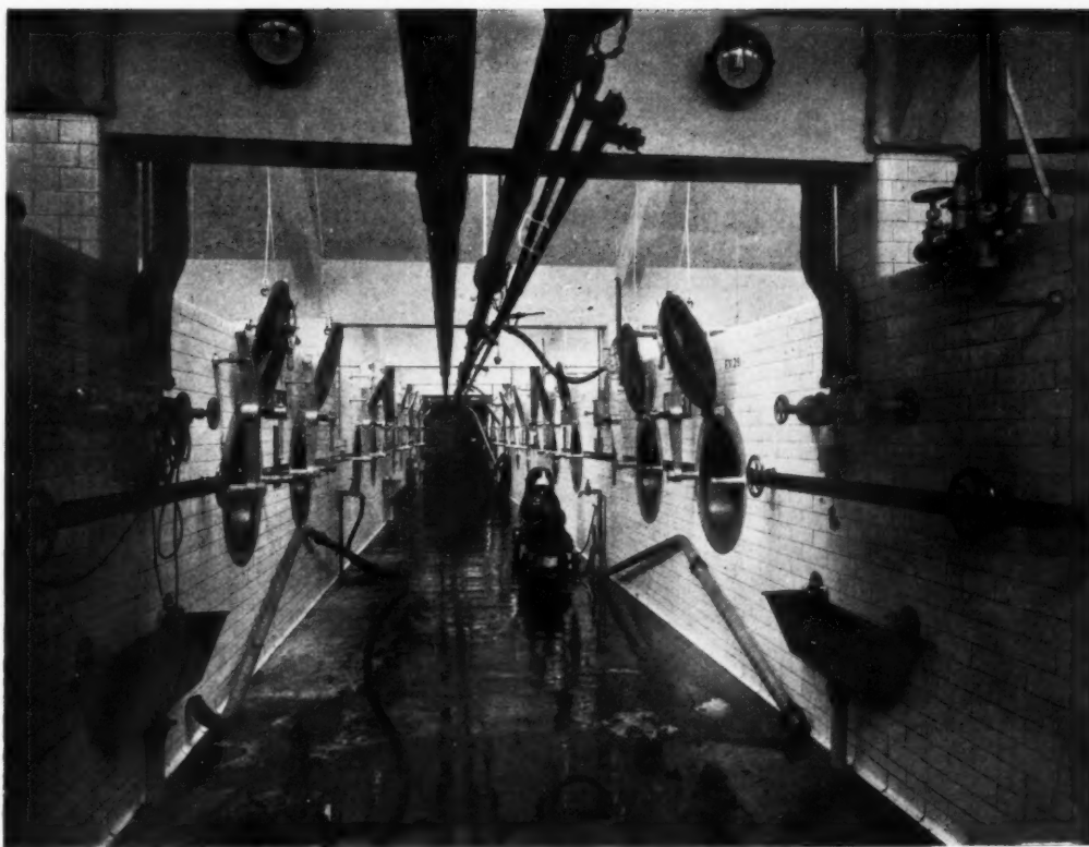
Messrs. Meux's Brewery, Nine Elms. Above, the concrete north-light roof over tuns ; below, the tun-room.
