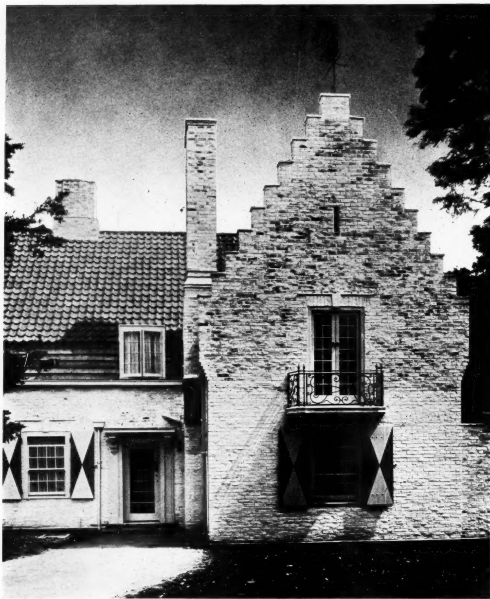
A house at Worthing (1924). The walls are of stock bricks, whitewashed, the roofs are covered with old pantiles, and the weatherboarding is oak.
