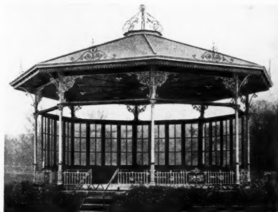
Bandstand at Luton, showing top rail for folding and sliding wind screens not reaching to the ceiling. Note how the effect might be improved by filling in above the head of the screen with treillage work to form a frieze.
