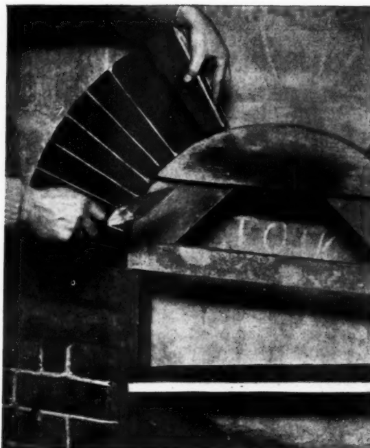
Figure two (left). The bricklayer's line is used in conjunction with the plumb-rule for the purpose of keeping the brickwork in plane vertical surfaces. Other factors in the production of plane surfaces are the porosity of the bricks and the composition of the mortar. Figure three (right). Trying the brick in position is a necessary preliminary to bedding it. Although every precaution has been taken to set out the brick geometrically in accordance with the full-size diagram, its actual appearance in the work is the real test.
