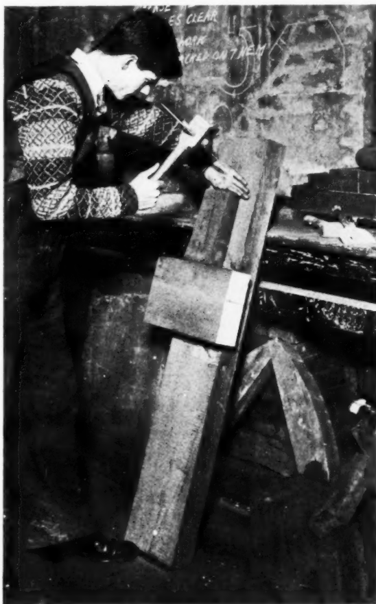
Figure six. Using the scutch. The brick is held with the left hand, and the plank supporting it is being kept steady with the left foot.
