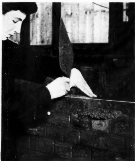
Figure two (left). The bricklayer's line is used in conjunction with the plumb-rule for the purpose of keeping the brickwork in plane vertical surfaces. Other factors in the production of plane surfaces are the porosity of the bricks and the composition of the mortar. Figure three (right). Trying the brick in position is a necessary preliminary to bedding it. Although every precaution has been taken to set out the brick geometrically in accordance with the full-size diagram, its actual appearance in the work is the real test.
