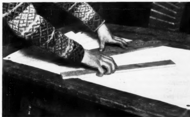
Figure four (left). Producing an absolutely true and flat bed by rubbing the brick on a stone after it has been cut approximately to shape by the brick-saw in the brick-cutting box. Figure five (right). The processes of marking the shapes upon the bricks are more lengthy and complicated than the architect would imagine. From the full-size drawing straight-edged and wedge-shaped wooden templates are made for use in the brick-cutting box or for scribing the outlines upon the faces of the bricks.
