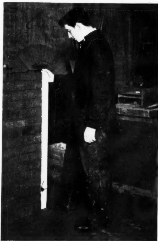
Figure one. Applying the plumb-rule to ensure that the end of the wall is being built in a vertical plane. Both hand and foot are used in keeping the plumb-rule pressed against the work.
