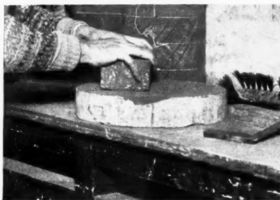
Figure four (left). Producing an absolutely true and flat bed by rubbing the brick on a stone after it has been cut approximately to shape by the brick-saw in the brick-cutting box. Figure five (right). The processes of marking the shapes upon the bricks are more lengthy and complicated than the architect would imagine. From the full-size drawing straight-edged and wedge-shaped wooden templates are made for use in the brick-cutting box or for scribing the outlines upon the faces of the bricks.
