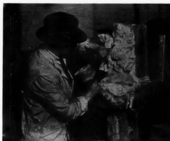
Left, figure three. Cutting an ornamental border upon a slab. The channels on the lower part of the slab show how the depth of background for the ornament is first settled. A chisel with the blade ground round at the corners is used to form the rounded hollows in the leaves. The chisel has a cup-shaped hollow in its driving end, whose edge bites into the soft iron head of the hammer. Right, figure four. Cutting an ornamental boss in a block of Portland stone with mallet-headed chisel and beechwood mallet. To support the block during the operation it is bedded against two heavier blocks with plaster of Paris.
