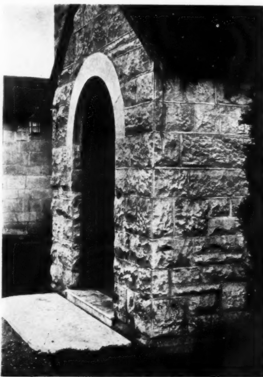
Above, figure five. Odd pieces from a stone contractor's yard have been utilized in this boundary wall. Rubbed texture is seen in the name plate, and sawn, boasted, hammer-dressed, and naturally-cleft surfaces may be recognized in the different fragments. Below, figure six. Portland stone porch. The smaller blocks are hammer-dressed on their faces, and the larger blocks are dressed with a hammer and with occasional blows with a "point." A small drafted margin is provided at the quoins to permit of the application of the plumb rule. The plinth is boasted, and the doorstep rubbed.
