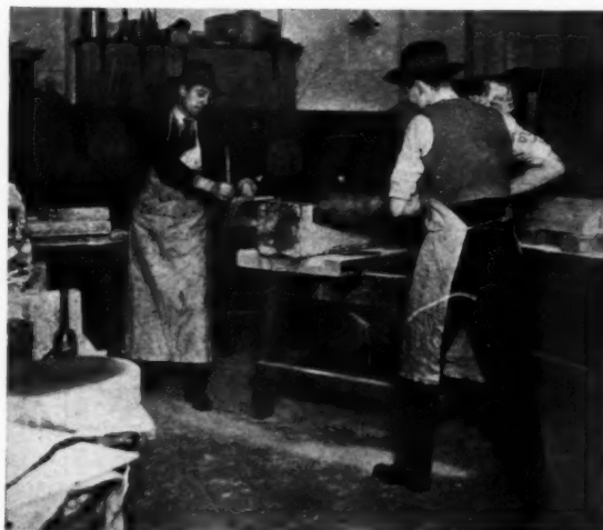
Figure one. Sawing a block of Portland stone to an exact length. The teeth of the saw in passing cut in either direction. They are given only a very slight set, and the cut is only slightly wider than the thickness of the saw blade.
